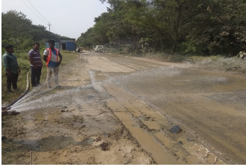
Photograph showing water sprinkling in haul road
